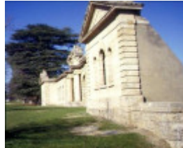
h00358 old hospital ruins church st beechworth view across facade she project 2003
