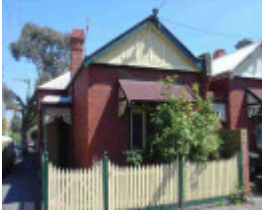
fitzroy north bennett street fitzroy north bennett street 15
