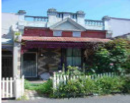
fitzroy north bennett street fitzroy north bennett street 37
