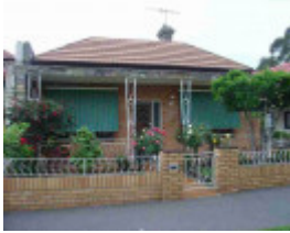
fitzroy north holden street fitzroy north holden street 30
