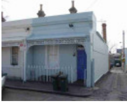
fitzroy moor street fitzroy moor street 85
