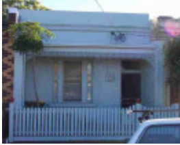
fitzroy north bennett street fitzroy north bennett street 75
