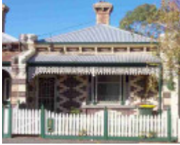
fitzroy north bennett street fitzroy north bennett street 76
