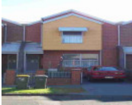
fitzroy north bennett street fitzroy north bennett street 111
