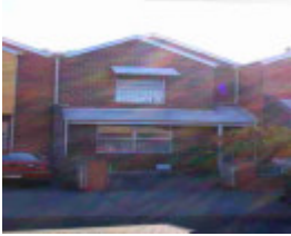
fitzroy north bennett street fitzroy north bennett street 113
