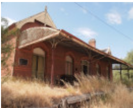
H1590 FORMER RUPANYUP RAILWAY STATION LHA 2015 2.JPG
