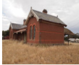
H1590 FORMER RUPANYUP RAILWAY STATION LHA 2015 1.JPG
