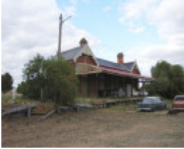
FORMER RUPANYUP RAILWAY STATION SOHE 2008
