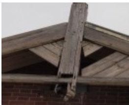
H1590 FORMER RUPANYUP RAILWAY STATION LHA 2015 5.JPG
