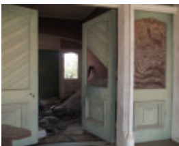
H1590 FORMER RUPANYUP RAILWAY STATION LHA 2015 8.JPG
