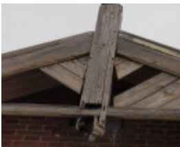
H1590 FORMER RUPANYUP RAILWAY STATION LHA 2015 5.JPG
