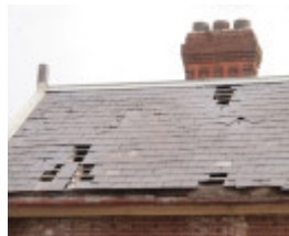
H1590 FORMER RUPANYUP RAILWAY STATION LHA 2015 4.JPG
