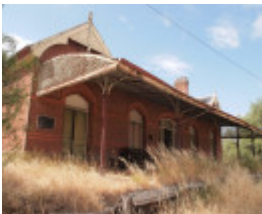
H1590 FORMER RUPANYUP RAILWAY STATION LHA 2015 2.JPG
