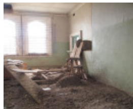
H1590 FORMER RUPANYUP RAILWAY STATION LHA 2015 7.JPG
