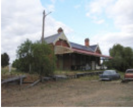
FORMER RUPANYUP RAILWAY STATION SOHE 2008
