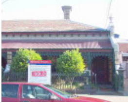
fitzroy north grant street fitzroy north grant street 3
