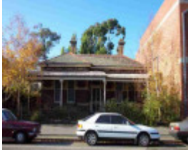
fitzroy north grant street fitzroy north grant street 8
