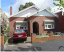
fitzroy north birkenhead street fitzroy north birkenhead street 51
