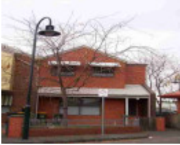
fitzroy north holden court fitzroy north holden court 4
