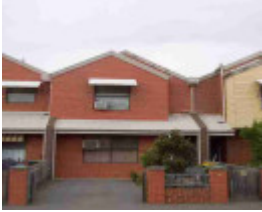
fitzroy north holden court fitzroy north holden court 8
