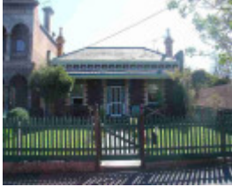
fitzroy north mckean street fitzroy north mckean street 153
