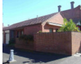
Fitzroy North Mckean Street 159-161.JPG
