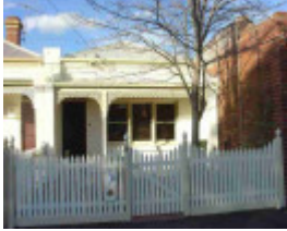
fitzroy north michael street fitzroy north michael street 86
