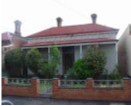
fitzroy north brunswick street fitzroy north brunswick street 843
