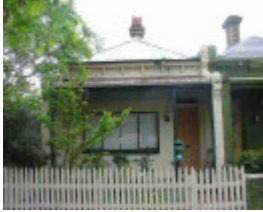
fitzroy north liverpool street fitzroy north liverpool street 17
