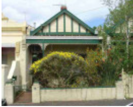
fitzroy north liverpool street fitzroy north liverpool street 20
