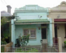
fitzroy north liverpool street fitzroy north liverpool street 21
