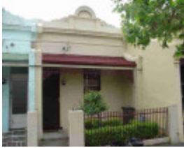
fitzroy north liverpool street fitzroy north liverpool street 23
