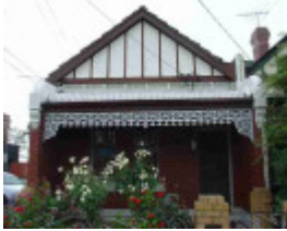
fitzroy north holden street fitzroy north holden street 62
