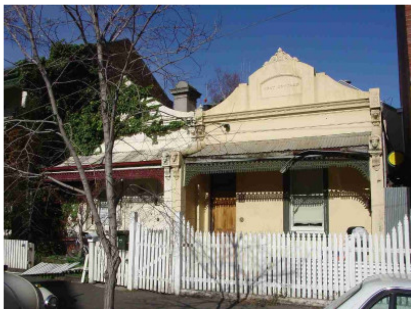
Fitzroy Victoria Street 112-114.JPG
