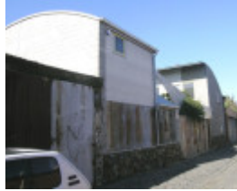
Rear of 29 Kneen Street.JPG
