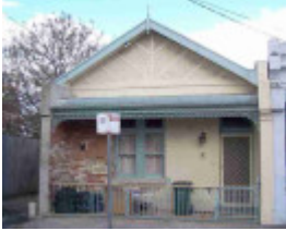
fitzroy north howe street fitzroy north howe street 8
