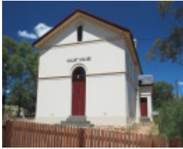
RUSHWORTH COURT HOUSE SOHE 2008
