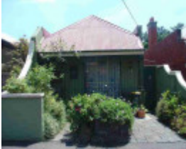
fitzroy north holden street fitzroy north holden street 233
