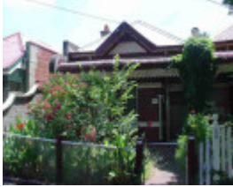
fitzroy north holden street fitzroy north holden street 235
