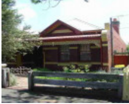
fitzroy north holden street fitzroy north holden street 241
