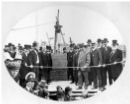
1909 - Laying of Grandstand Foundation Stone
