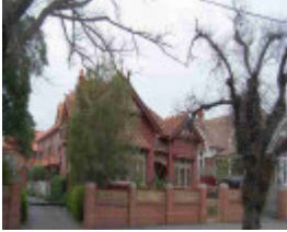
fitzroy north queens parade fitzroy north queens parade 240 unit 3
