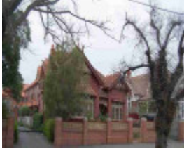
fitzroy north queens parade fitzroy north queens parade 240 unit 7
