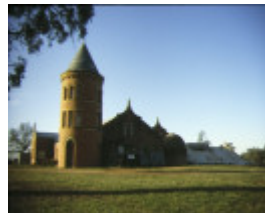
1 mount ophir winery stillards lane rutherglen view of winery jun1981
