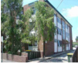
fitzroy north barkly street fitzroy north barkly street 262 unit 1
