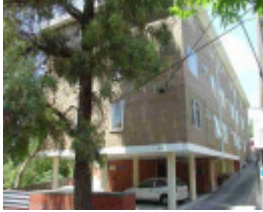
fitzroy north barkly street fitzroy north barkly street 272 unit 1-18
