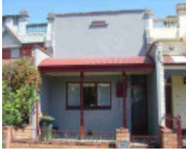
fitzroy north bennett street fitzroy north bennett street 39
