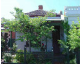
fitzroy north bennett street fitzroy north bennett street 40
