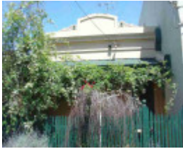
fitzroy north church street fitzroy north church street 58
