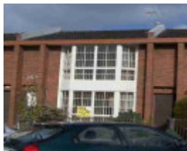
carlton north fenwick street carlton north fenwick street 95 unit 2
