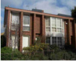
carlton north fenwick street carlton north fenwick street 95 unit 3
