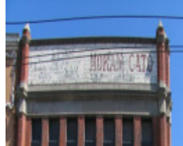
moran and cato fading signage.jpg
