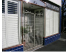
Shopfront - 97 Delbridge Street
