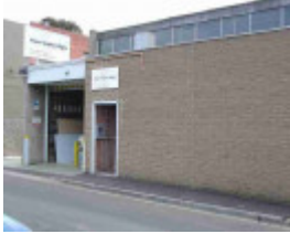
fitzroy rose street fitzroy rose street 45-53 unit 1
