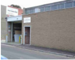
fitzroy rose street fitzroy rose street 45-53 unit 1
