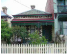
fitzroy north rushall crescent fitzroy north rushall crescent 8
