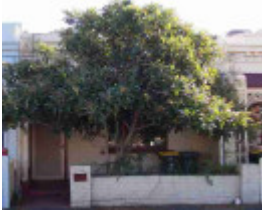
fitzroy north bennett street fitzroy north bennett street 77
