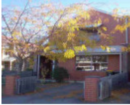
fitzroy north bennett street fitzroy north bennett street 95
