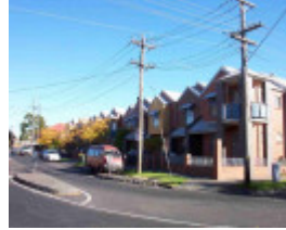
Fitzroy North Bennett Street 95-115.JPG
