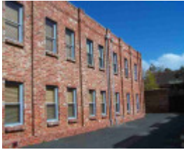
fitzroy north mckean street fitzroy north mckean street 274b
