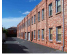
Fitzroy North Mckean Street 274.JPG
