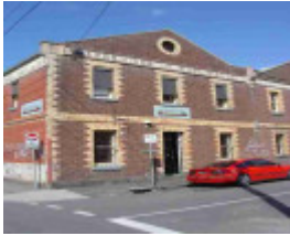
fitzroy spring street fitzroy spring street 12
